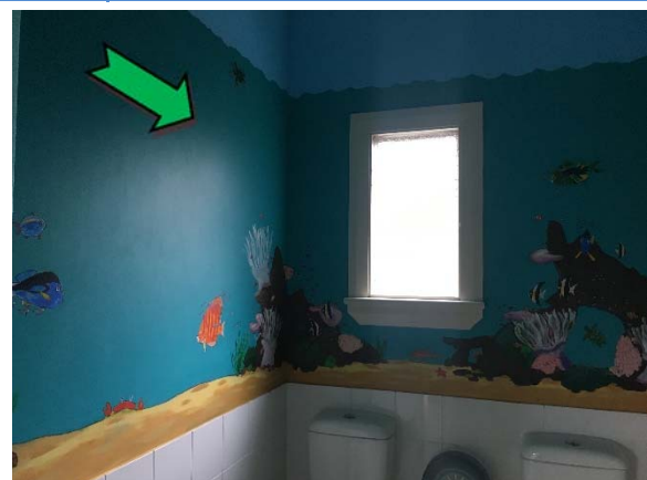
Photo 6. Interior, bathroom, walls – non asbestos-containing fibre cement sheeting.
