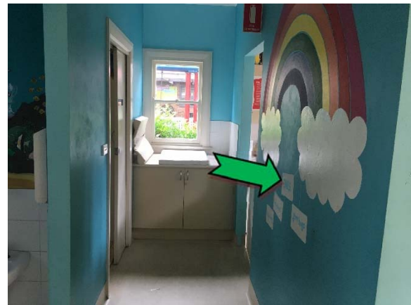
Photo 4. Interior, east corridor, walls – non asbestos-containing fibre cement sheeting.
