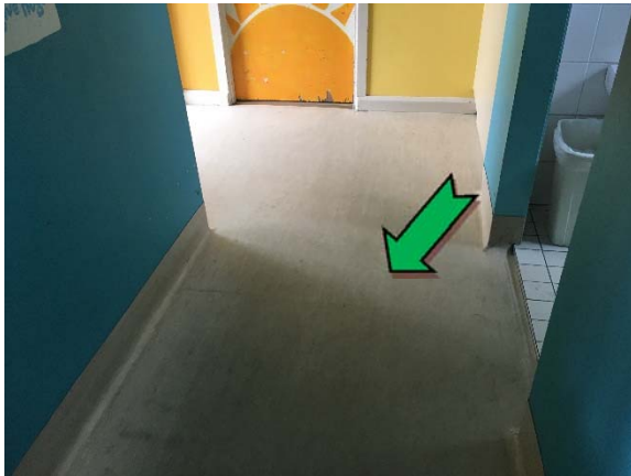
Photo 9. Interior, throughout, floor coverings – non asbestos-containing sheet vinyl.
