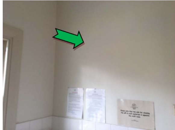
Photo 8. Interior, kitchen, walls – non asbestos-containing fibre cement sheeting.
