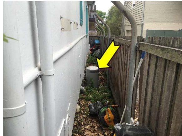
Photo 10. Exterior, western elevation, hot water heater – suspected SMF internal insulation material.
