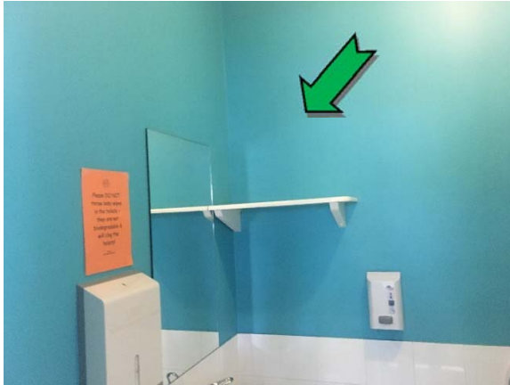
Photo 7. Interior, disabled toilet, walls – non asbestos-containing fibre cement sheeting.
