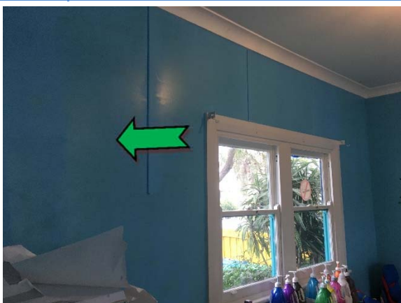
Photo 5. Interior, play room, walls – suspected non asbestos-containing material.
