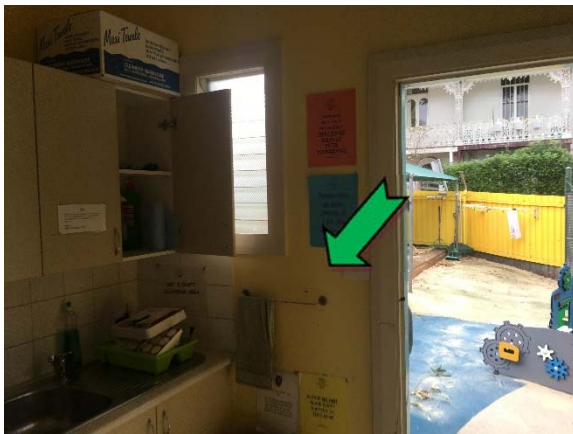
Photo 3. Interior, kitchen, walls – non asbestos-containing fibre cement sheeting.
